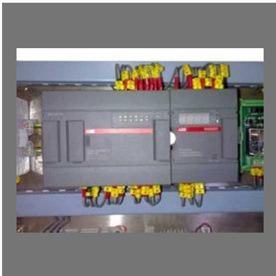
PLC Automation Control Panel
